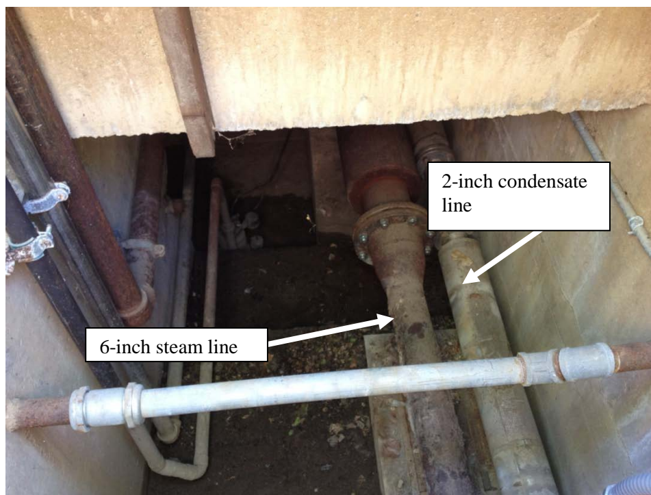
Figure 5: Utility corridor showing steam supply and condensate return lines
