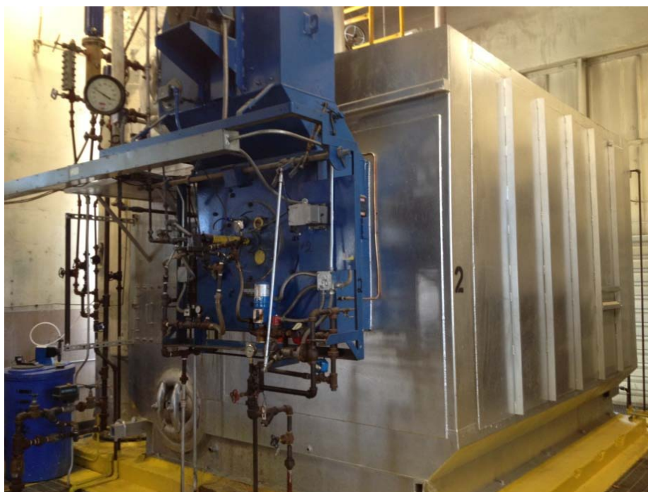
Figure 2: Boiler #2, 500 Horsepower Nebraska
