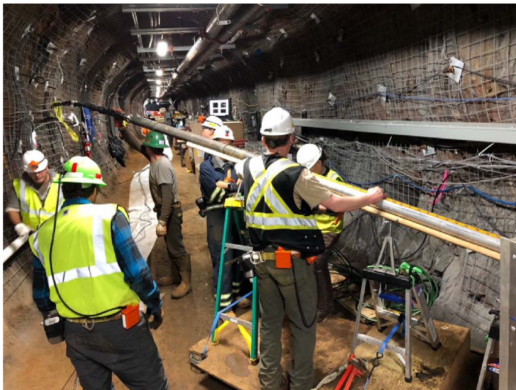
Figure 1: Removal of downhole instrumentation from production well (E1-P).
