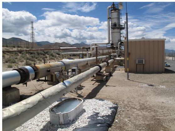
Figure 7. Fluid sampling sites, Roosevelt Hot Springs: A) mini-separator on a two-phase line, upstream of the separator, with steam jetting from the gas port; B) pipeline downstream of a separator with a drip tank containing cooled thermal water.
