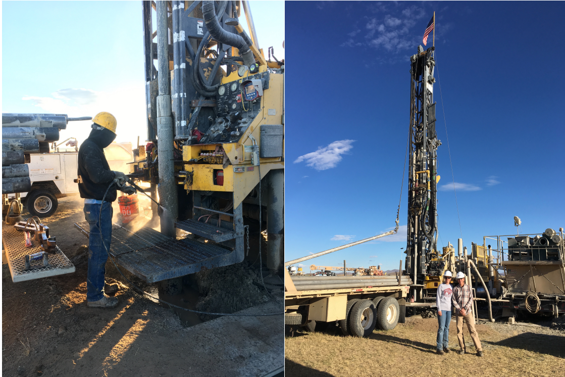
(Left) Washing of stabilizer (Right) Alex and Eric visiting the site.
