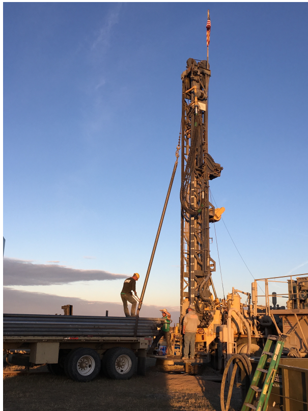
Tripping out at the end of the day.
