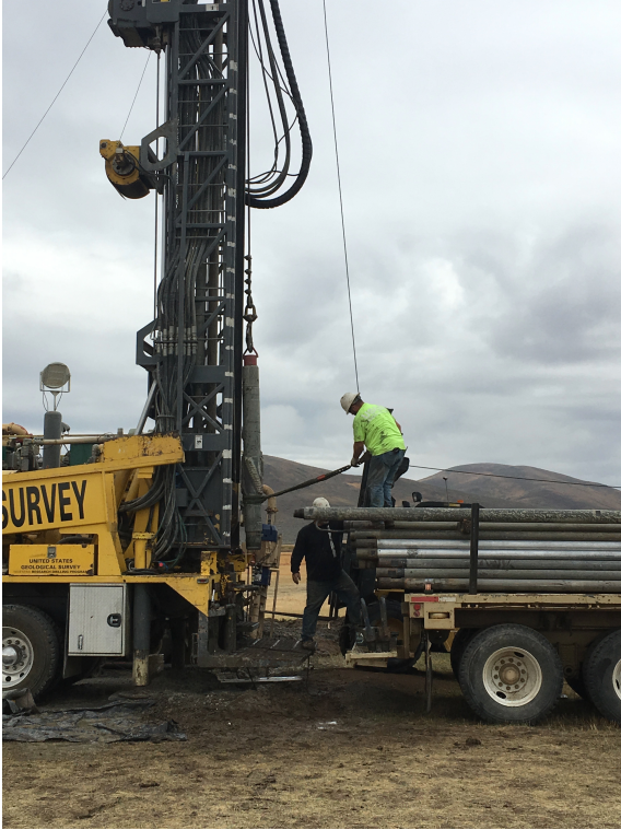
(Left) Removing stabilizer (Right) New drill bit and collar.
