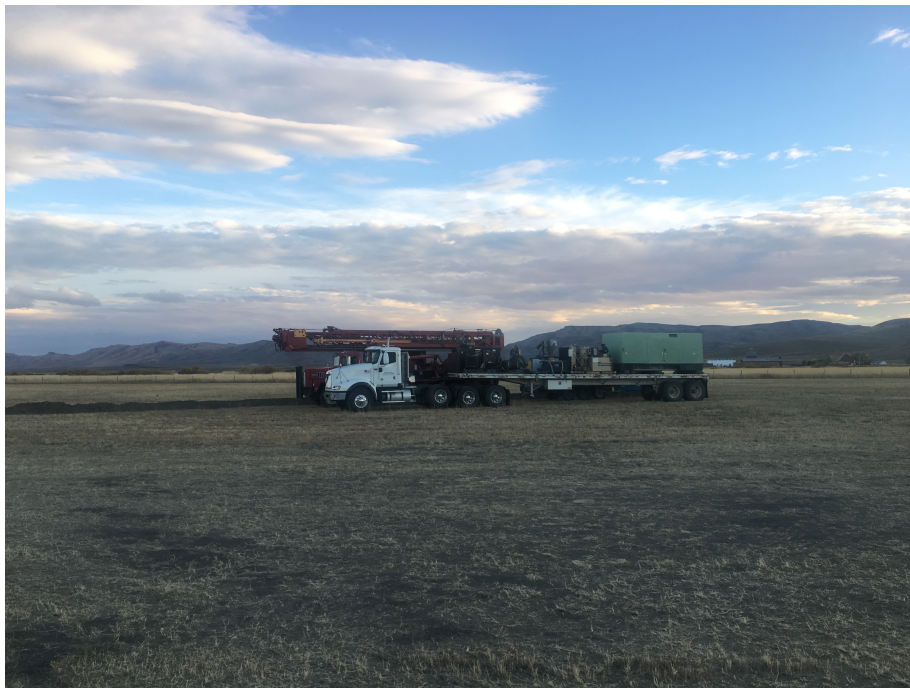
Arrival of new drill rig.
