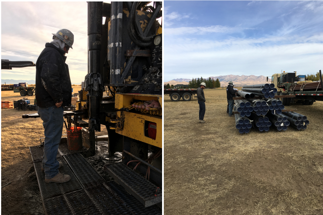
(Left) Inspecting the reaming bit assembly after cleaning. (Right) New casing.
