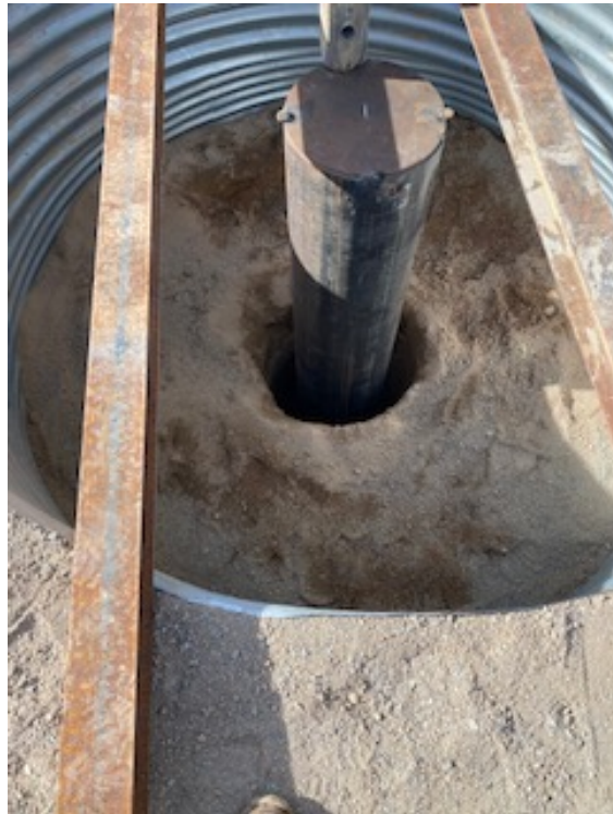
Figure 9: 20 in. conductor pipe
