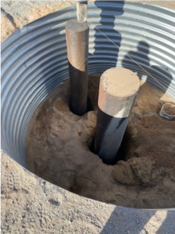
Figure 10: Conductor and mouse hole
