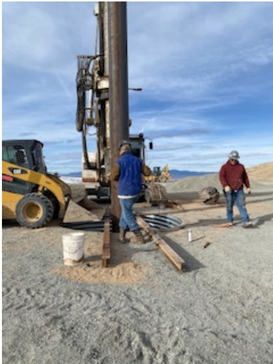
Figure 8: 56-32 cellar construction
