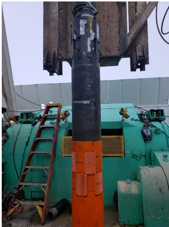
Figure 65. Photograph of a portion of the liner hanger assembly before running in the hole.
