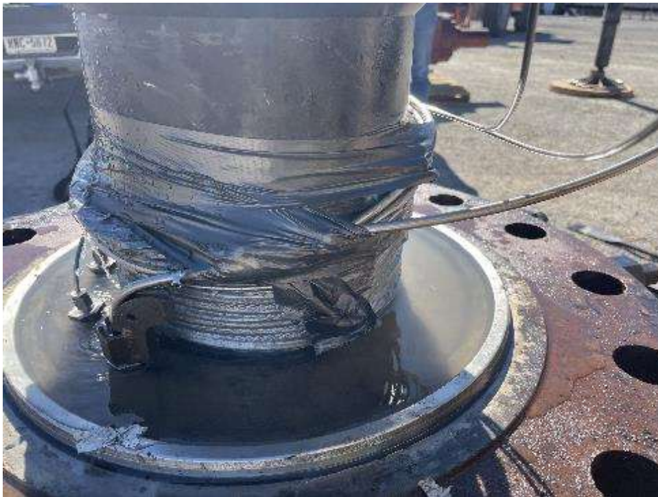
Figure 20. Fiber optic cables after Silixa removed three wraps (during wellhead repair).
