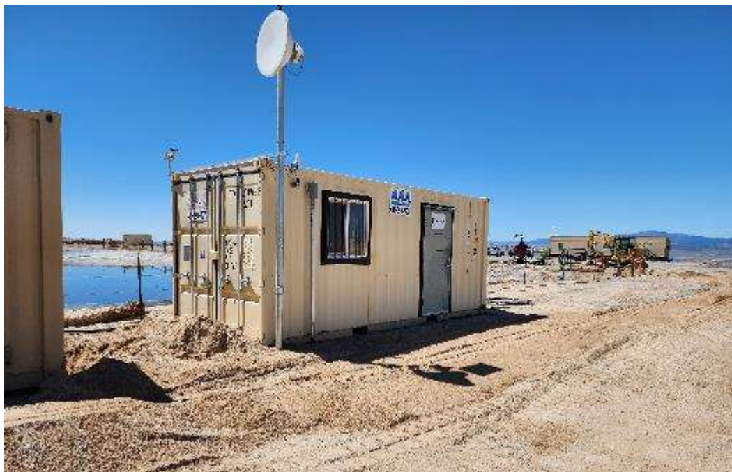
Figure 18. Silixa acquisition trailer after trench has been backfilled.
