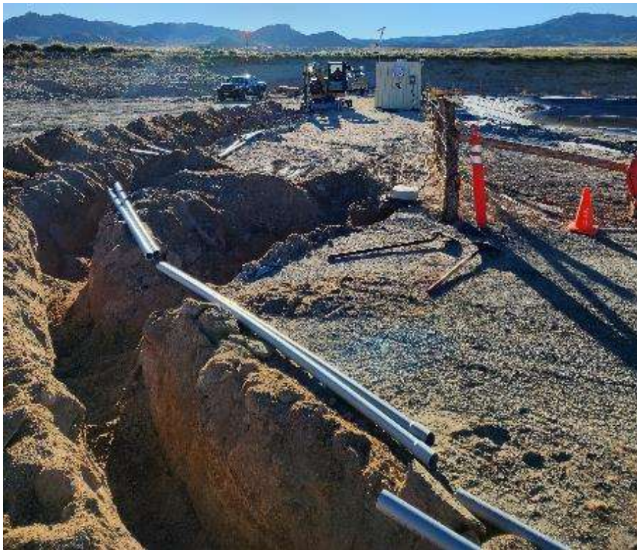
Figure 16. Conduit trenching from enclosure frame to acquisition trailer.
