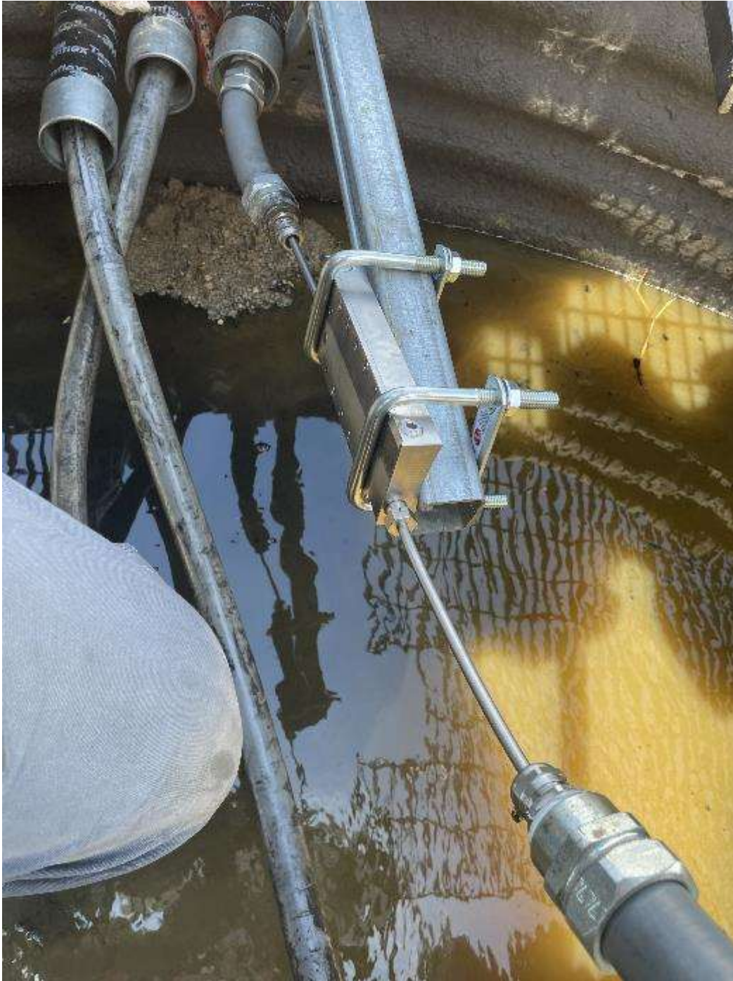
Figure 23. In-line repair splice located underneath 16B cellar grating.
