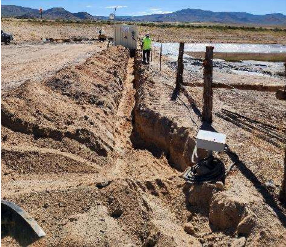
Figure 19. Trenching for permanent trailer electrical supply.
