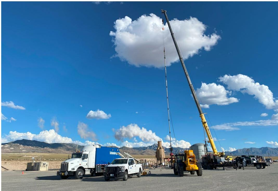
**Figure 5-10:** Utah FORGE Well 16B test site with lubricator stacks for chemical tool.
