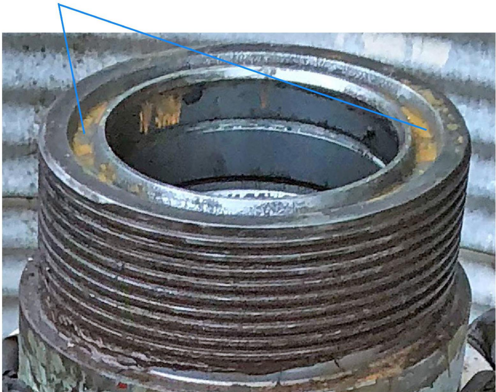
Figure 37 General Corrosion of Ring Groove
