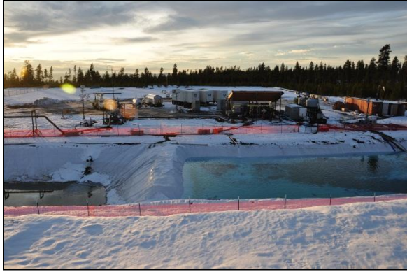
Figure 2: Newberry stimulation site photo. Showing from right to left, booster pump system, stimulation pump, high-pressure piping, TZIM injection system, wellhead assembly, and flowtesting set-up
