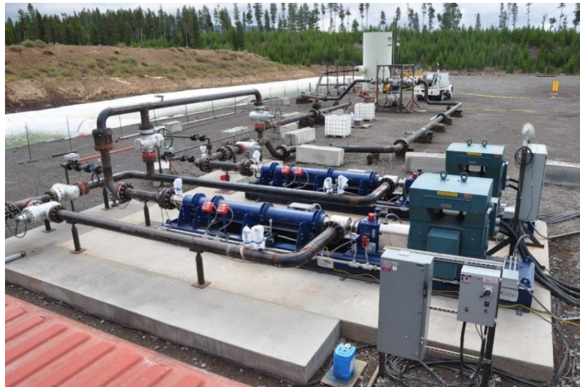
Figure 2: Horizontal, centrifugal pumps (blue), electric drives (green), and 10" (OD) piping to well head in the background.
