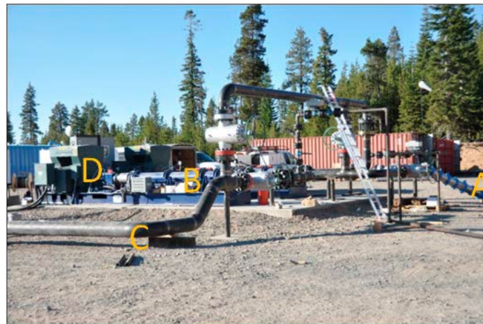
Figure 4. Newberry stimulation site photo. Shown from right to left, A. low pressure inlet (silver pipe with blue joints), B. stimulation pumps (blue), C. high-pressure piping, and D. variable speed drives (green).
